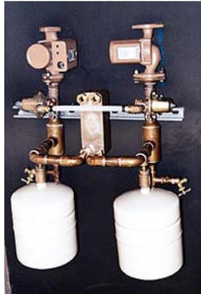
*SuperStor's Voyager water heater works well in dual-purpose applications, for both drinking water and space heating. Voyager offers a built-in heat exchanger, but the author prefers to use an external unit, shown preassembled with expansion tanks and circulators in the photo (above left). The heat exchanger is fully insulated and is located between the tank and the red and blue heating loop manifold (above right).*
