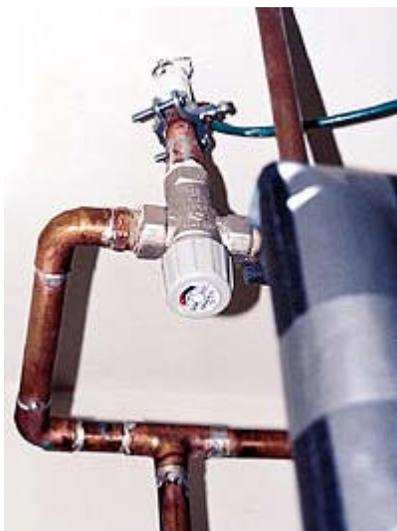
*Figure 6. When water heaters are used for both space heating and domestic water, the domestic side must usually be mixed with cold water for safety's sake. A mechanical tempering valve is a simple way to do this.*
