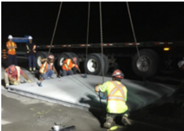
Placement of panels during overnight construction
