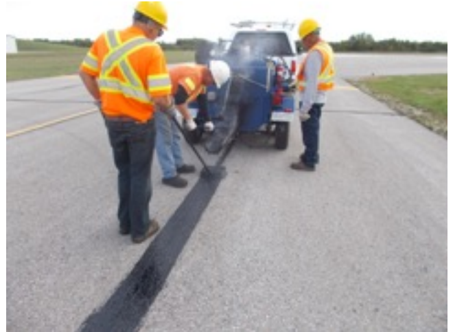
Figure 2. Kettle with agitator used to heat the product to the discharge temperature and a box used to guide the material into the cracks
