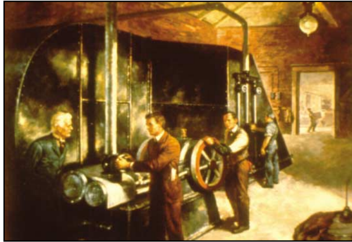
First air-conditioning plant at Brooklyn, N.Y., printing company.
