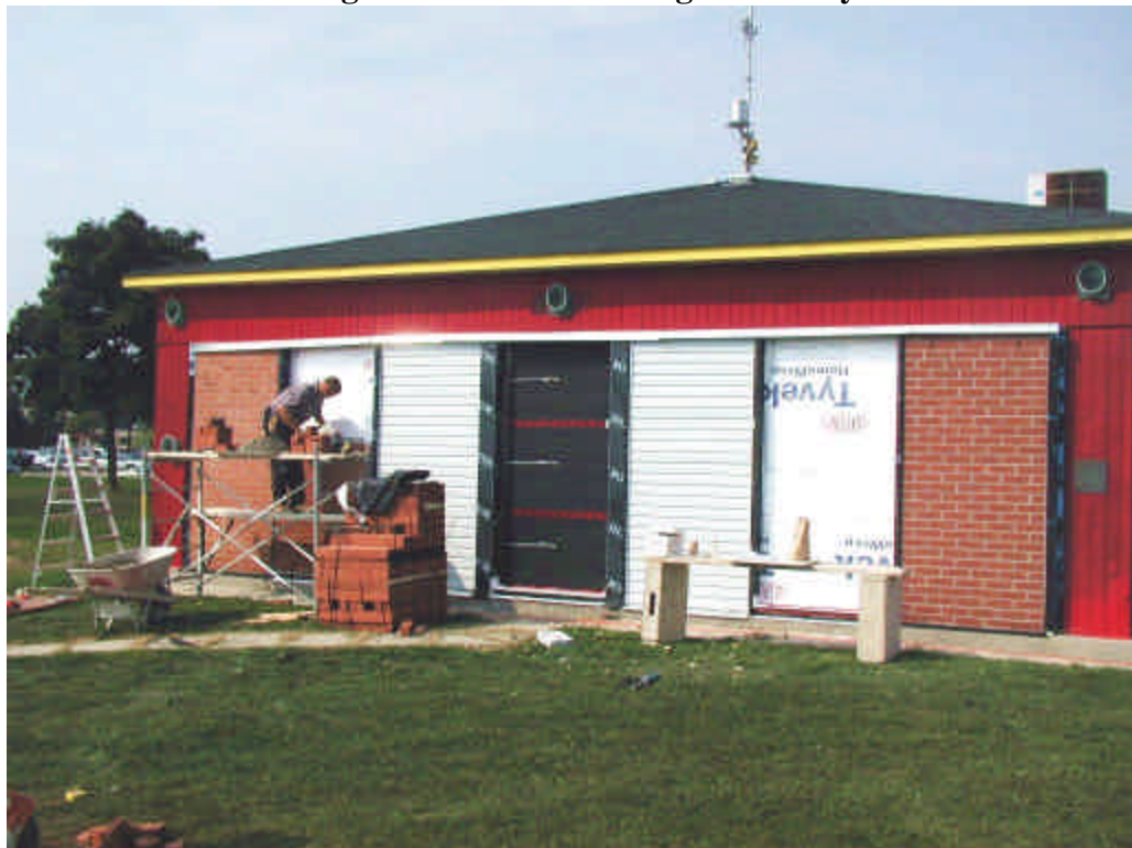
Masons Install a Brick Veneer after Instrumented Panels are Installed
