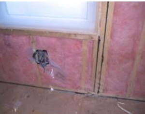
Poly can be (?) an air and vapour barrier
