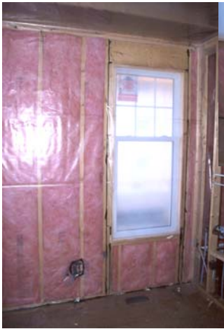
Poly can be (?) an air and vapour barrier
