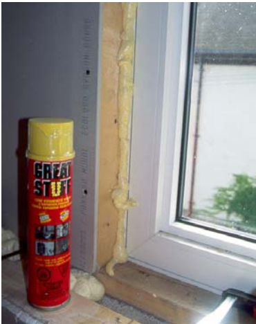
Air sealing around windows and other openings
