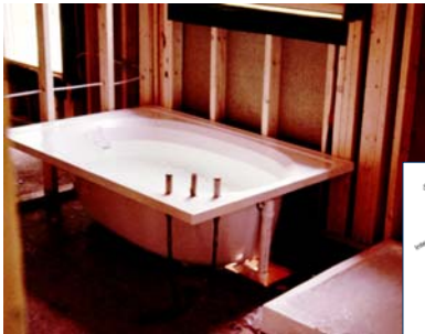
Big Air Leakage Points
