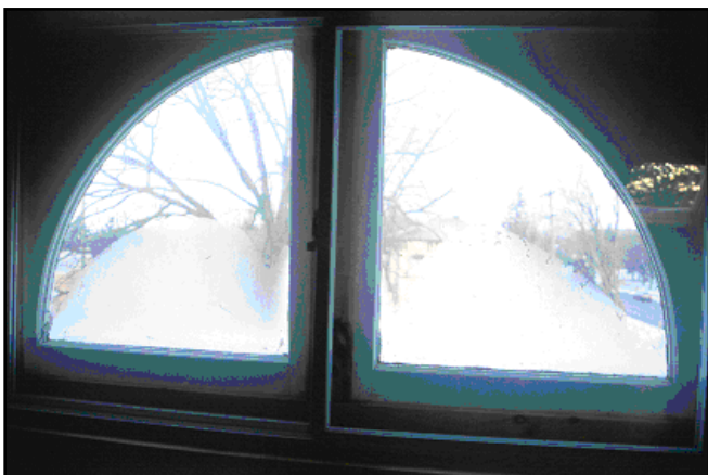
Water vapor has bypassed the vapor impermeable interior glazing unit (by convection through small flaws in the caulking) and condensing on the exterior pane of this window in winter. The same phenomena occur within walls and roofs as in the wall at right.
