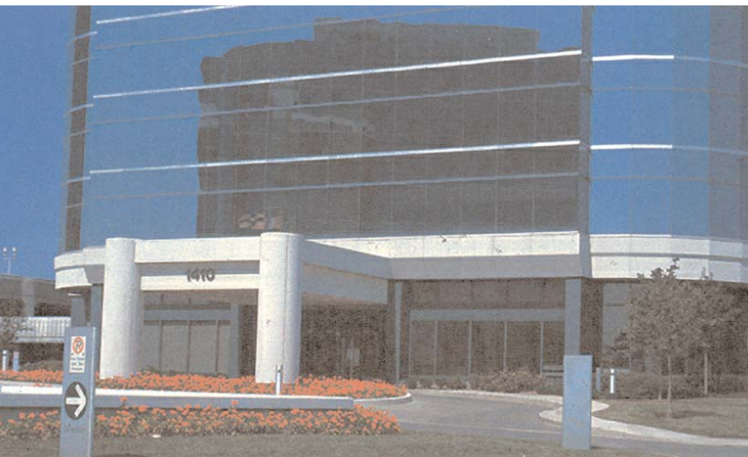
Fig. 6 – Structural Silicone Glazing System
