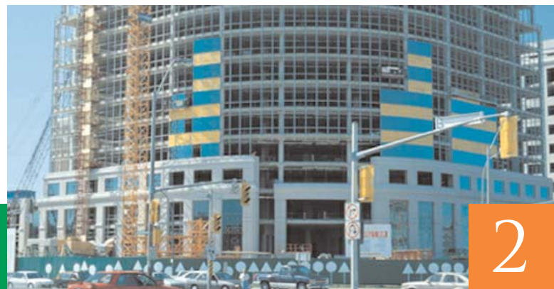
Fig. 2 – Stick Built Curtain Wall System – Ottawa Post Office
