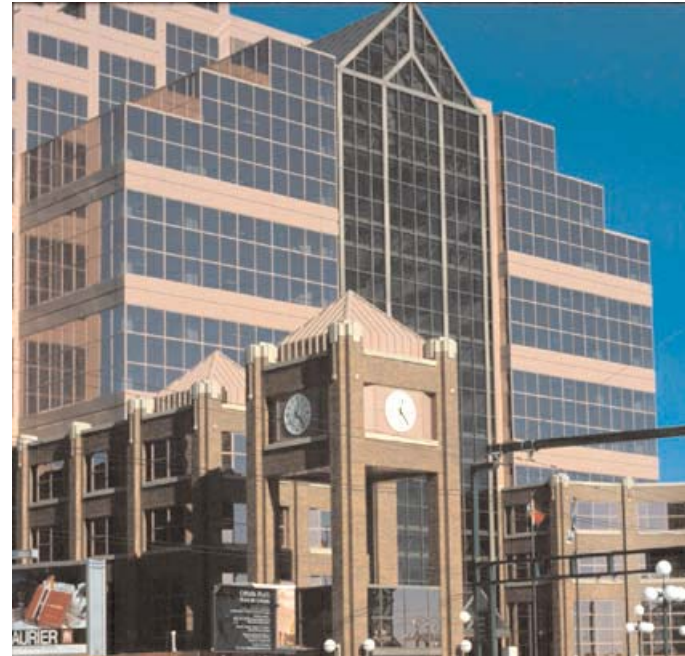
Fig. 1 Curtain Wall With Granite Spandrel Panels
