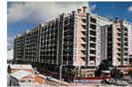
Photo: Courtesy of Arup Eastgate, a large office block in Harare, Zimbabwe, relies on long, narrow floor plates for maximum daylighting and ventilation.
