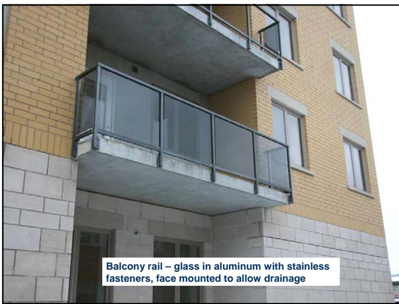
Balcony rail – glass in aluminum with stainless fasteners, face mounted to allow drainage
