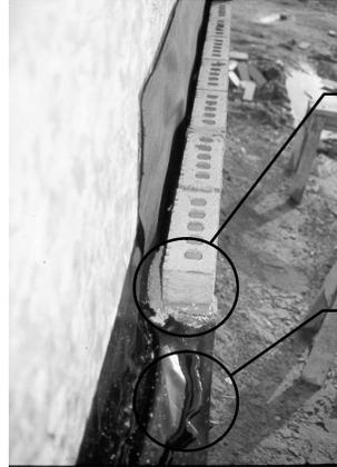
Water can build up here -- we need a waterproof barrier
