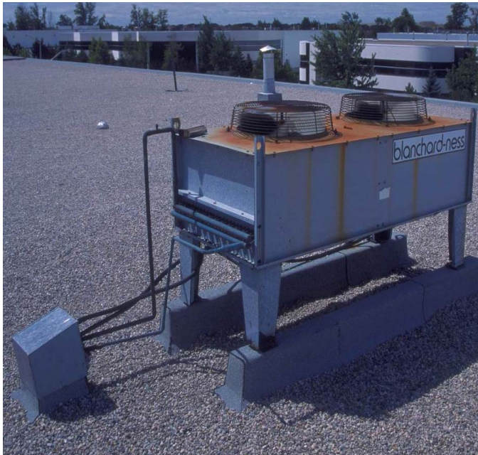
A pair of DX heat rejection devices (note refrigerant lines) for small loads
