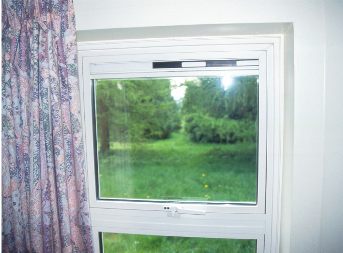
A British Window with a trickle ventilator at the head
