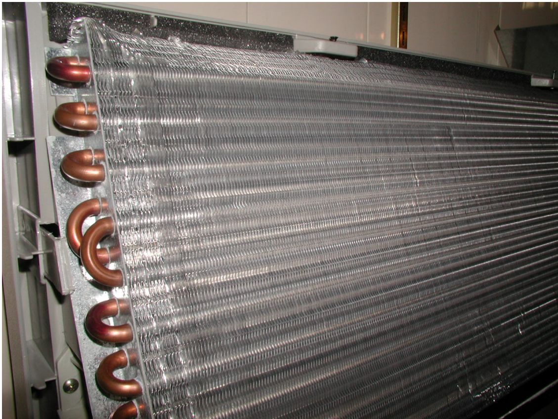
A view of a finned coil heat exchanger within a residential cooling system. It contains refrigerant that boils away at about 5 C / 40 F and takes heat with it.
